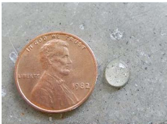
FIG. 1 Non-absorptive Concrete Surface
